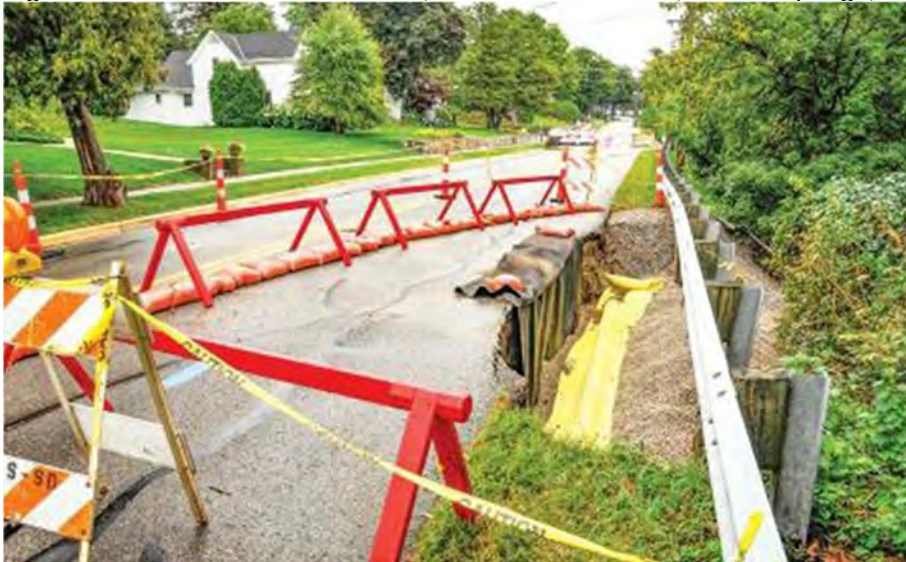
Figure 17. Washout Area on M-119, near Harrison Street, Harbor Springs, September 2022
