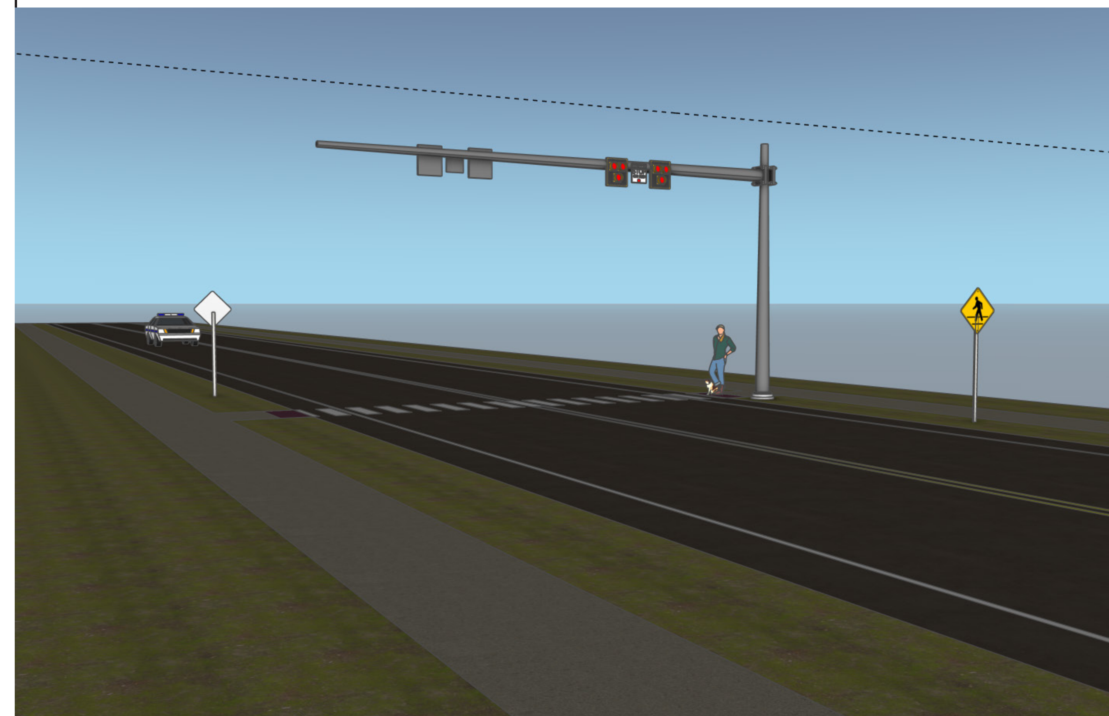
High-intensity Activated crossWALK (HAWK) signal.
