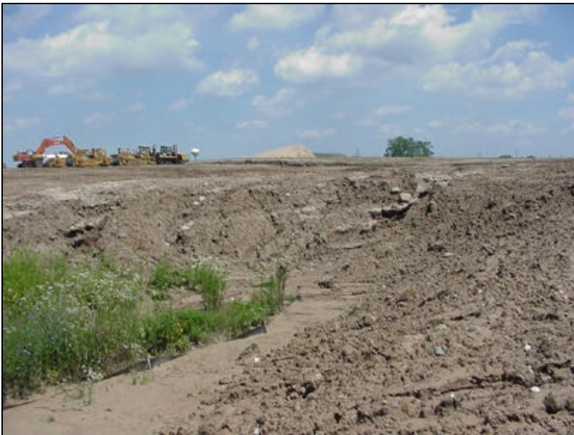
Development projects leave soil prone to erosion. Notice the failing silt fence near the vegetation. Photo: Ottawa County SESC Agency.
