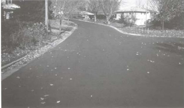
The picture in the upper left shows a newly constructed road which would be given a rating of 10. The upper right picture shows a recent overlay making this road a rating of 9. The picture to the left would be rated an 8 because a recent slurry seal was applied. Similarly the picture in the bottom right corner had a chip seal put down giving the road surface a rating of 8. The picture in the bottom left corner would also be rated an 8 for its surface which needs almost no maintenance. Notice the widely spaced sealed cracks.
