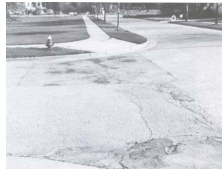
The pictures below show road surfaces with ratings of 2 and 1. Examples of defects from rating 2 include rutting greater than 2", patches in very poor condition, and extensive alligator cracking. Surface defects for a rating of 1 include: extensive loss of surface, numerous potholes, and severe alligator cracking.
