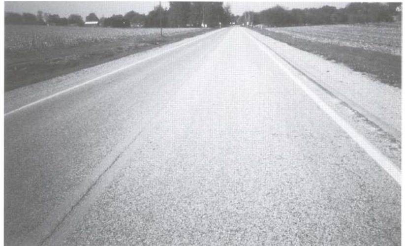
Ratings of 5-7 require capital preventative maintenance. These are roads that are beginning to show the first signs of wear. The roads are still structurally supported, but the surface may be starting to deteriorate. Capital preventative maintenance fixes protect the pavement structure and slow the rate of deterioration, which maintains and improves the functional condition of the road. The photographs below show roads in the capital preventative maintenance category.
