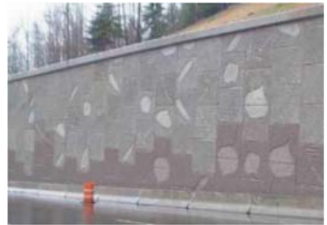
Broad leaf pattern on noise wall at the Sunset Interchange on I-90 in Issaquah.
