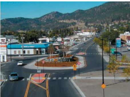
Finished roundabout in Colville.
