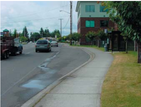
Bus pullout at transit stop in Tumwater.
