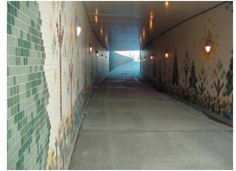
A bike tunnel in Lacey.
