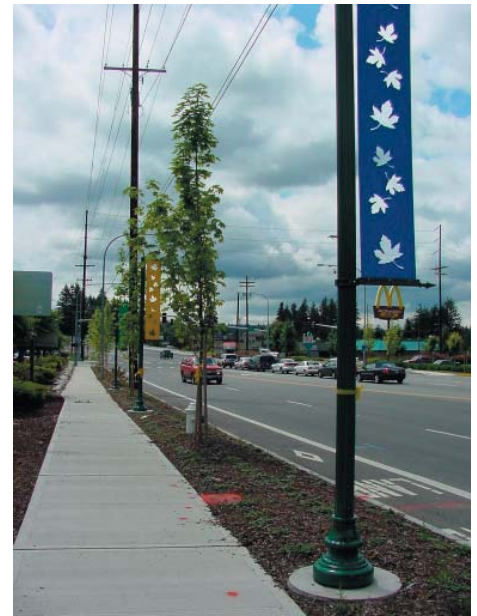
Multifunction roadway on SR 169 in Maple Valley.
