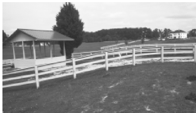
This small, attractive shed functions as a state-of-the-art manure processing facility, converting fresh stable sweepings into dry usable compost in two short weeks.
