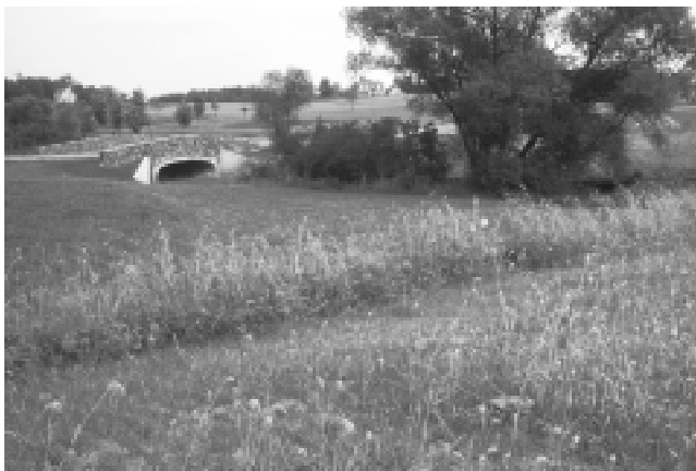
Riparian vegetation was both preserved and enhanced (with native specie plantings) along the Dobbins Creek Greenway, pictured here with a low-impact bridge faced with local stone. Note also the gravel roadway, whose rougher surface serves to calm traffic speed and to reduce stormwater runoff.
