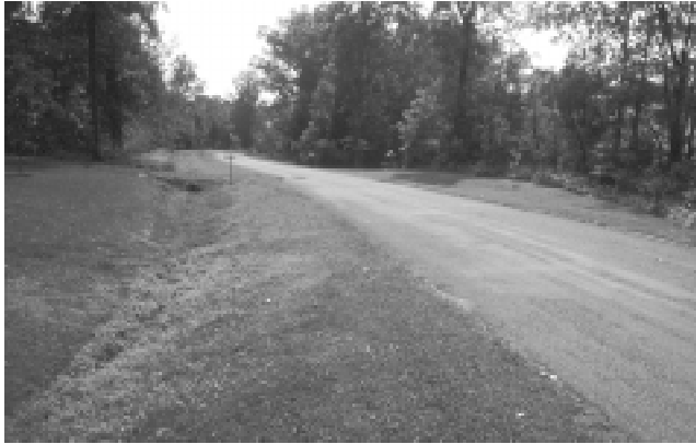
The subdivision street design at Cardinal Meadows utilizes open drainage swales rather than curbs, gutters and catch basins, enhancing the opportunity for on-site infiltration and groundwater recharge. Homes are screened from view on their private wooded lots.
