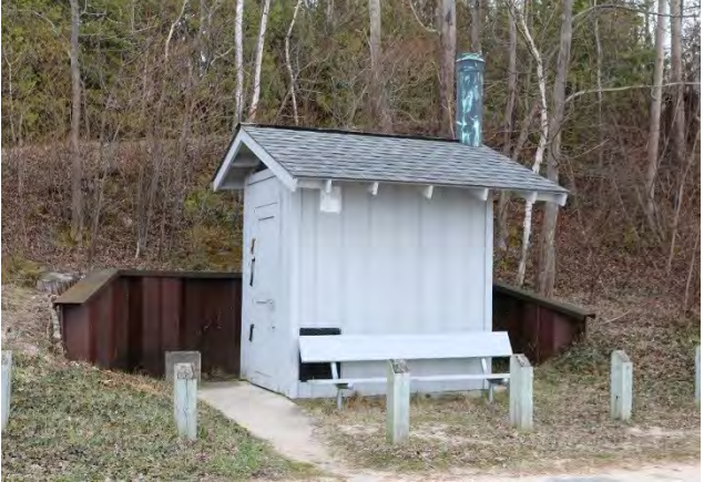
Vault Toilet off of the Parking Lot
