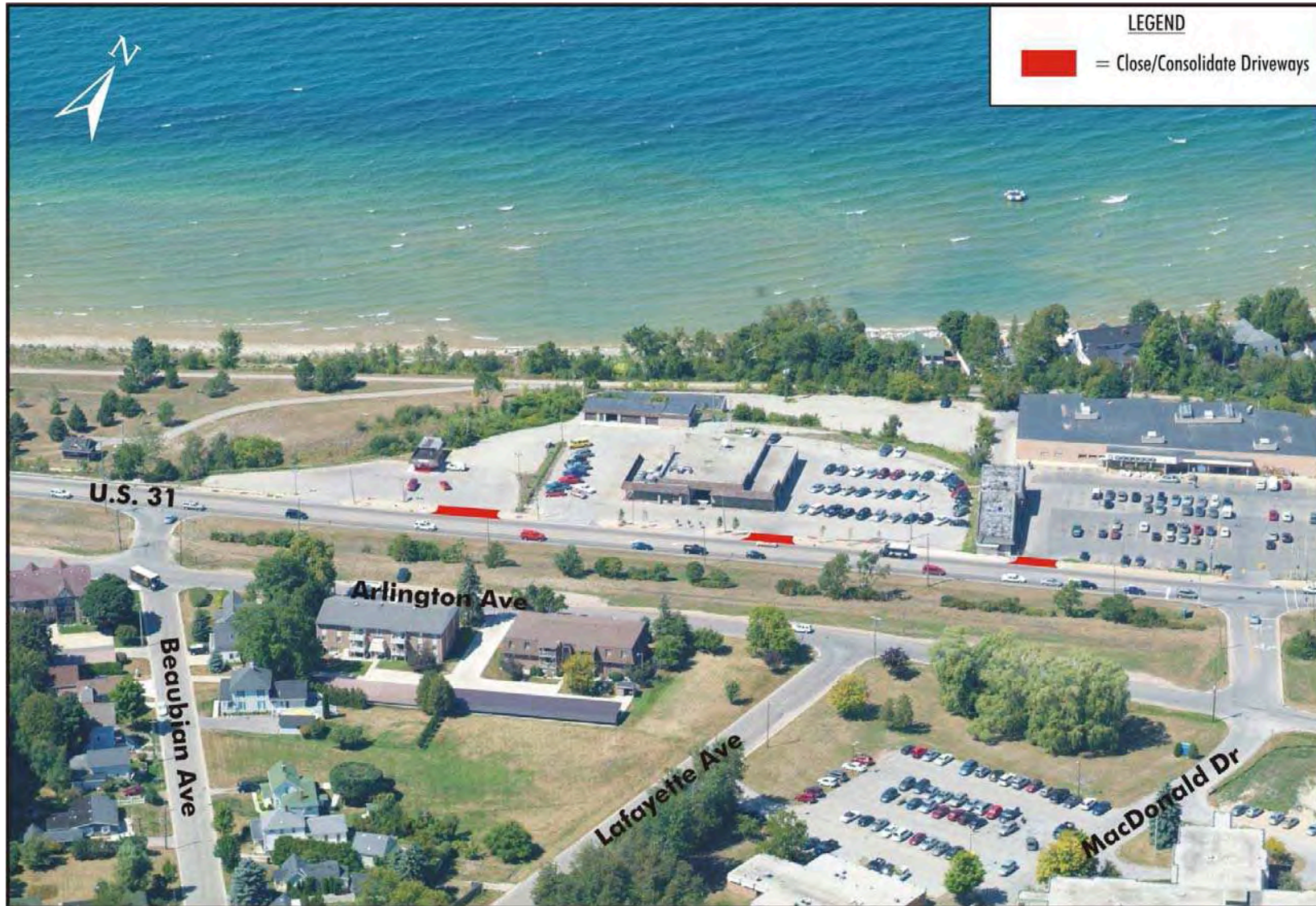
Figure 3-26 Petoskey Area-wide Transportation Concepts Access Management Concepts in Area of U.S. 31 between Beaubian and Lafayette Avenues
