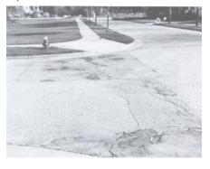
The pictures below show road surfaces with ratings of 2 and 1. Examples of defects from rating 2 include rutting greater than 2", patches in very poor condition, and extensive alligator cracking. Surface defects for a rating of 1 include: extensive loss of surface, numerous potholes, and severe alligator cracking.
