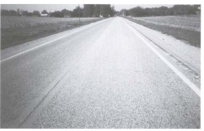
Ratings of 5-7 require capital preventative maintenance. These are roads that are beginning to show the first signs of wear. The roads are still structurally supported, but the surface may be starting to deteriorate. Capital preventative maintenance fixes protect the pavement structure and slow the rate of deterioration, which maintains and improves the functional condition of the road. The photographs below show roads in the capital preventative maintenance category.
